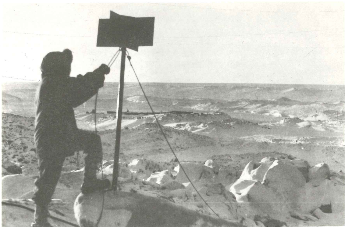
Plate 6 Erecting the beacon on G11, Casey triangulation survey, July 1975.
