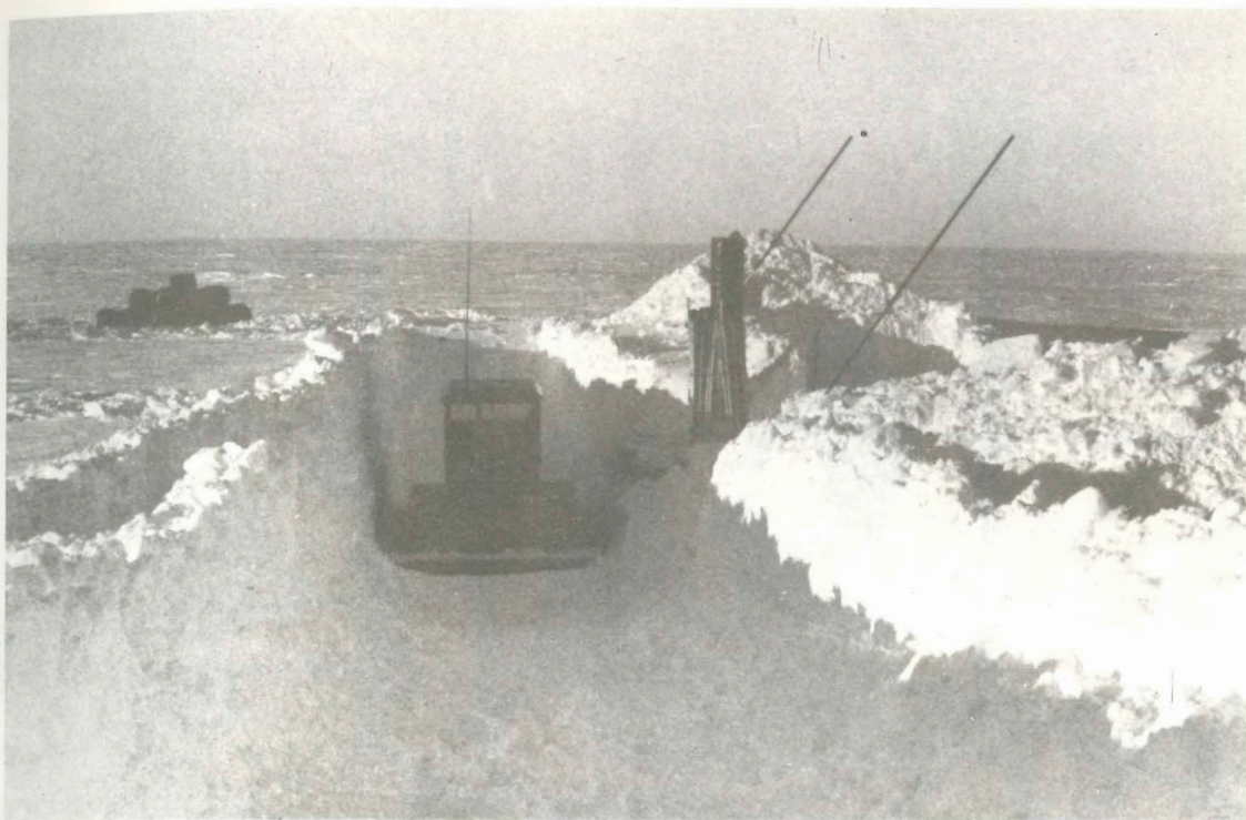
Plate 16 Excavating the 1973 fuel dump at A034 December 1975. The new dump is being re-established on the present surface level to the left in the photo.
