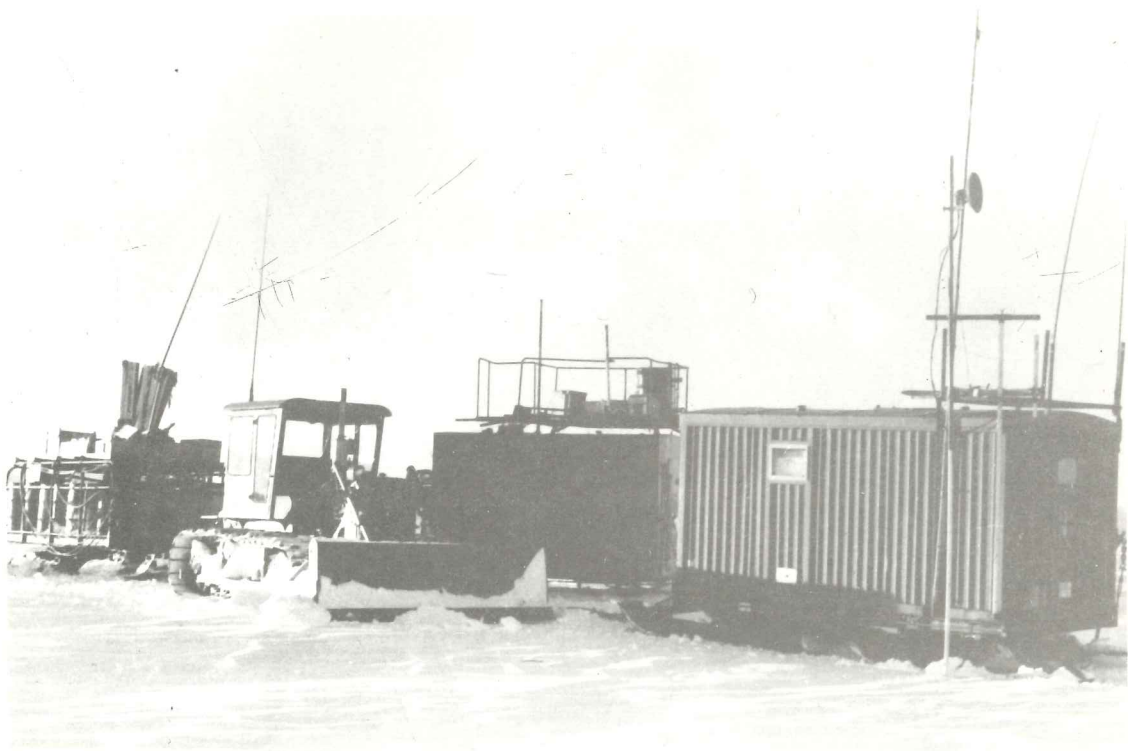
Plate 12 Tellurometer measurements in progress—note the antenna on the snowpole, the pole itself being clamped to the caravan.
